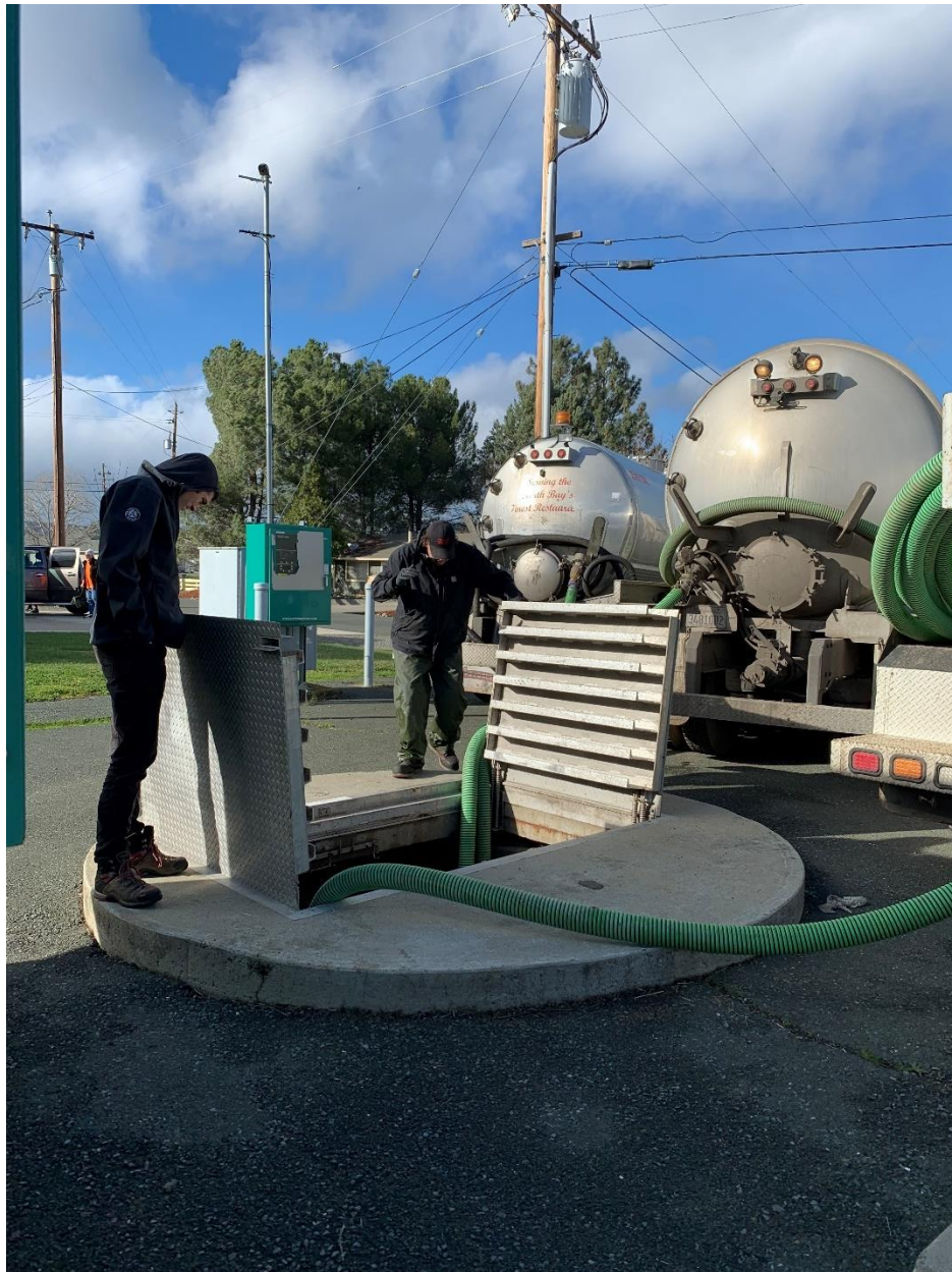
Figure 4-89 HVLCSD – Pumping and Hauling Operations
