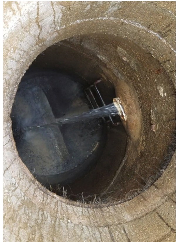
Manhole Inspections: Heavy flow from Deer Hill— North Shore easement
