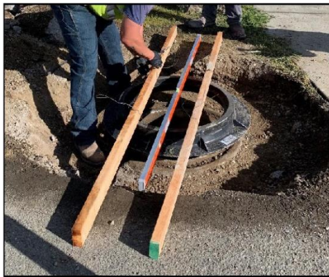
Figure 2: 2x4's to grade new manhole ring
