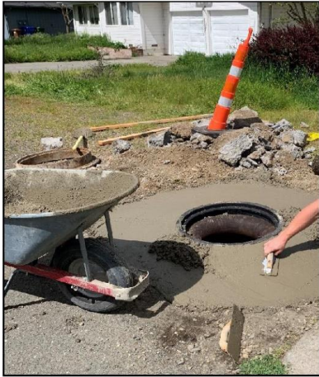
Figure 4: Even out the poured concrete
