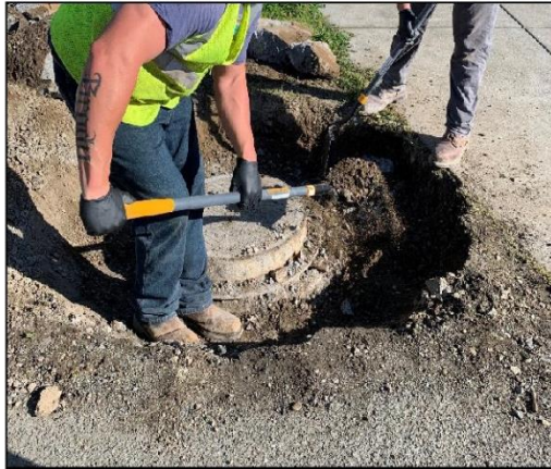
Figure 1: Concrete debris removal
