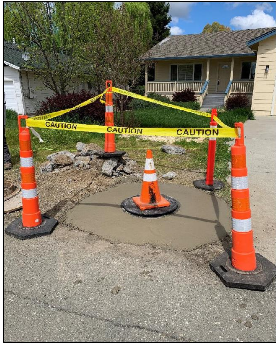
Figure 5: Manhole completion with safety cones and caution tape
