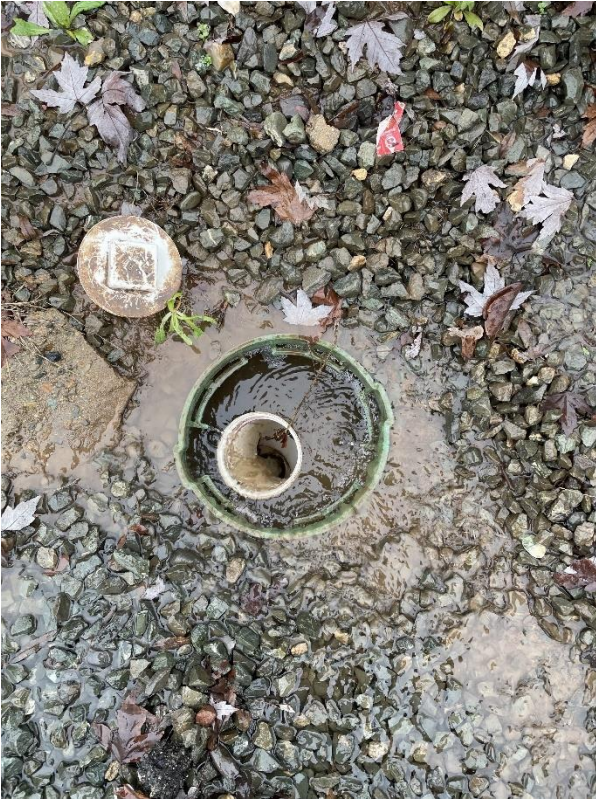
Figure 5: Residential cleanouts opened to reduce flooding on residential property.
