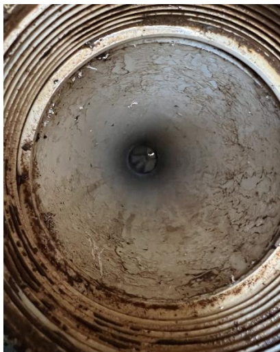
Cleanout repair from the residential cleanout.
